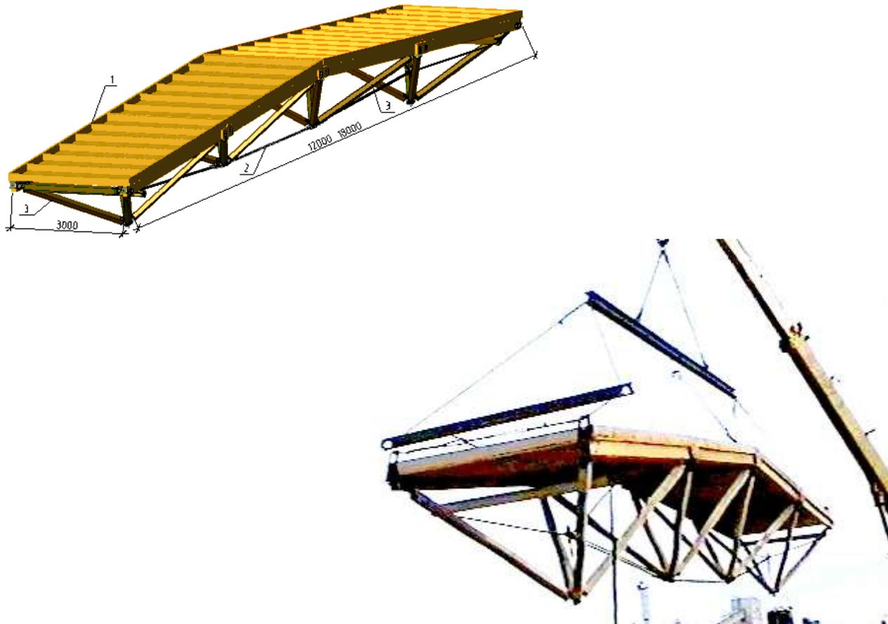
Fig. 8. Three-edged wood metal truss unit
